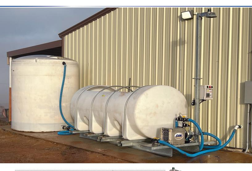
GVM's **Brine Production Systems** (BPS) are designed to convert dry rock salt into liquid for pre-wetting or anti-icing roadways. The use of salt brine lowers the freezing point of snow and ice and is popular and cost effective solution for managing roadways. GVM's Brine Production System lowers operation costs by using readily available materials; granular salt and tap water. They are capable of producing up to 5,000 gallons of brine per hour, depending on the water source.
